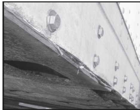
Fig. 22: Swelling Between Fasteners
